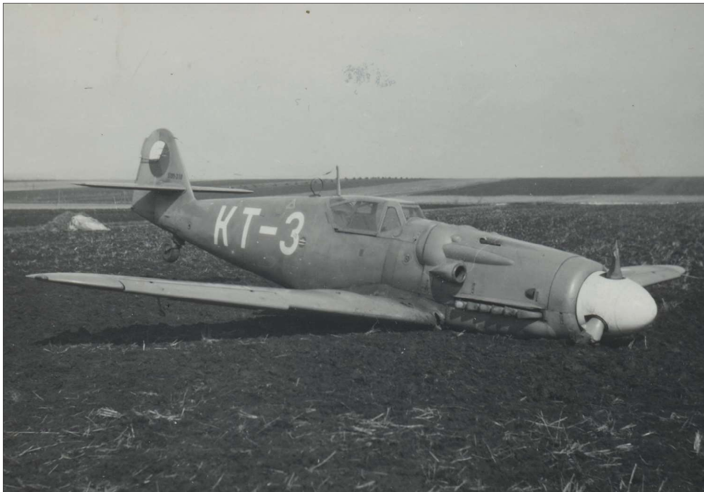
Aero produced S-199.310. On May 30, 1949, this airplane, coded KT-3, made a forced landing not far from Boskovice while flown by Lt. (Sgt) Karel Kessler. The code places the aircraft in the service of the 3rd Flight of the Air Regiment 7. This S-199 was only armed with the synchronized 131/13N fuselage machine guns, lacking the wing gun pods. After necessary repairs, the aircraft was updated with the rearward sliding bubble canopy and was equipped with reconnaissance equipment and reassigned to LP 1. In 1951, it served with the 5 Air Training Regiment in Zvolen, where it was coded UL-51 and obtained yellow training bands. It was likely that the reconnaissance equipment had been removed by that time.
